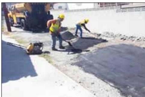
Recently, the city's Street Services Divison repaired the alley between 15th and 16th streets north of Patton Avenue. The two-person crew under the supervision of Street Services supervisor Hans Duran placed three tons of asphalt and smoothed out the pavement. The work was done as part of the city's small asphalt repair program in which neighborhood councils are asked to identify problem areas.
